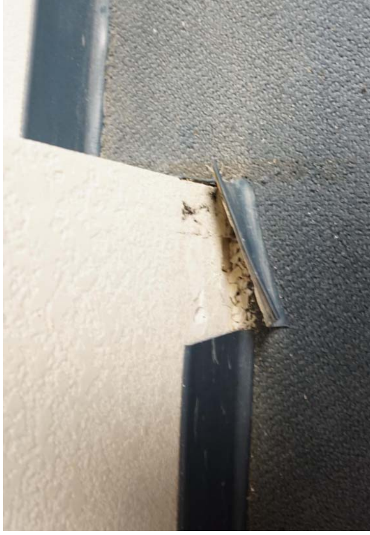
Room 145, NW corner, mold growth on wall at column
