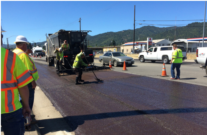
County crews add a seal coat to a roadway in Redwood Valley.
