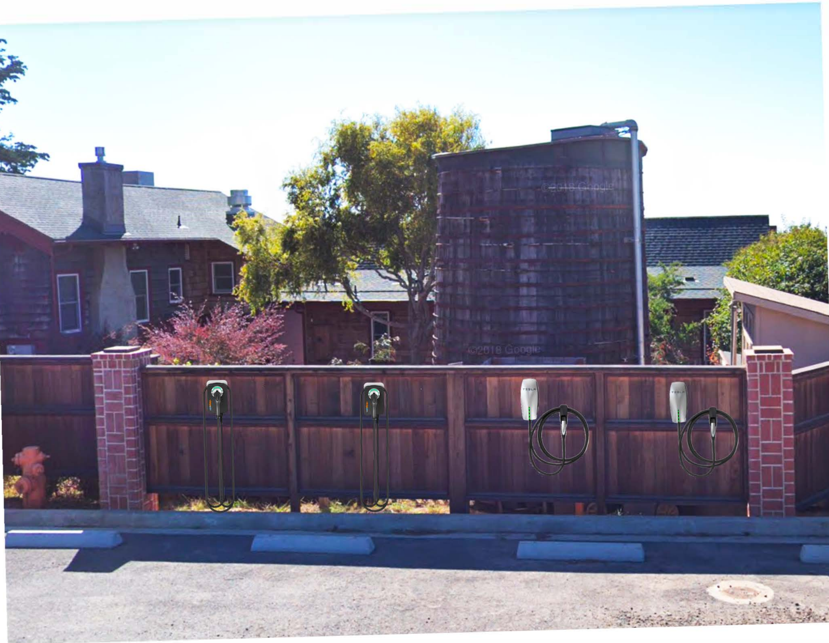
Proposed electric vehicle destination charging stations (four); to be installed on existing perimeter fence adjacent to parking spaces.
