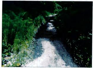
UNMAINTAINED IN-BOARD DITCH CAUSING WATER TO FLOW OVER TRAIL SURFACE
