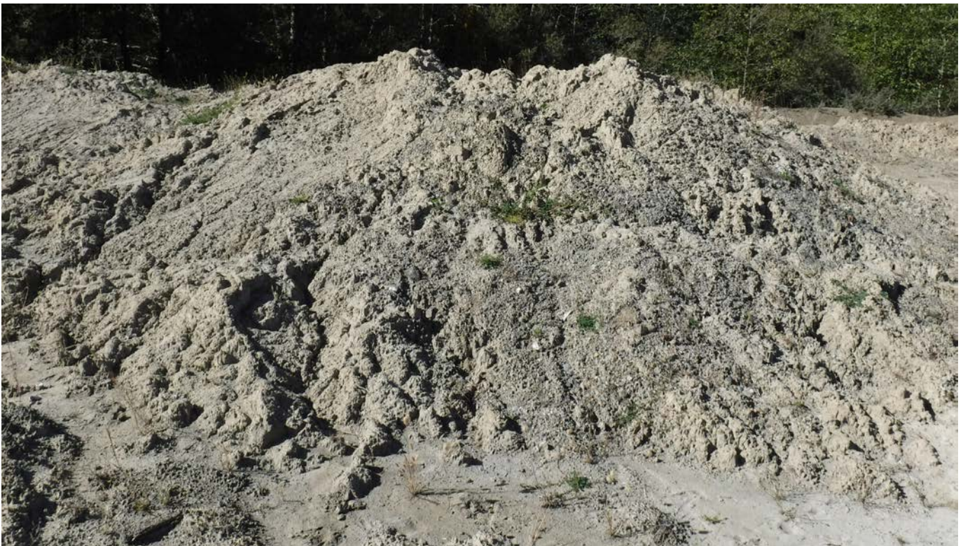
Photo #6 - Stockpiled sediments removed from sediment settling pond observed at pond's perimeter. As discussed in Sections VIII-5 and IX, it was recommended to spread hay on it. Compare with post-inspection photos by operator dated 11/20/2018.
