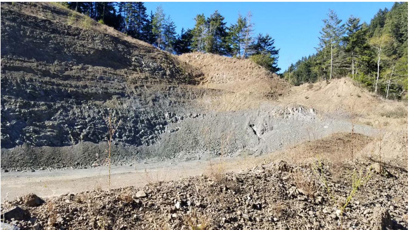
Photo #2 - View from quarry floor, looking west. Details on lower face slopes and mounds to be re-contoured on the right shown. Aggregate stockpile at the bottom of the picture.
