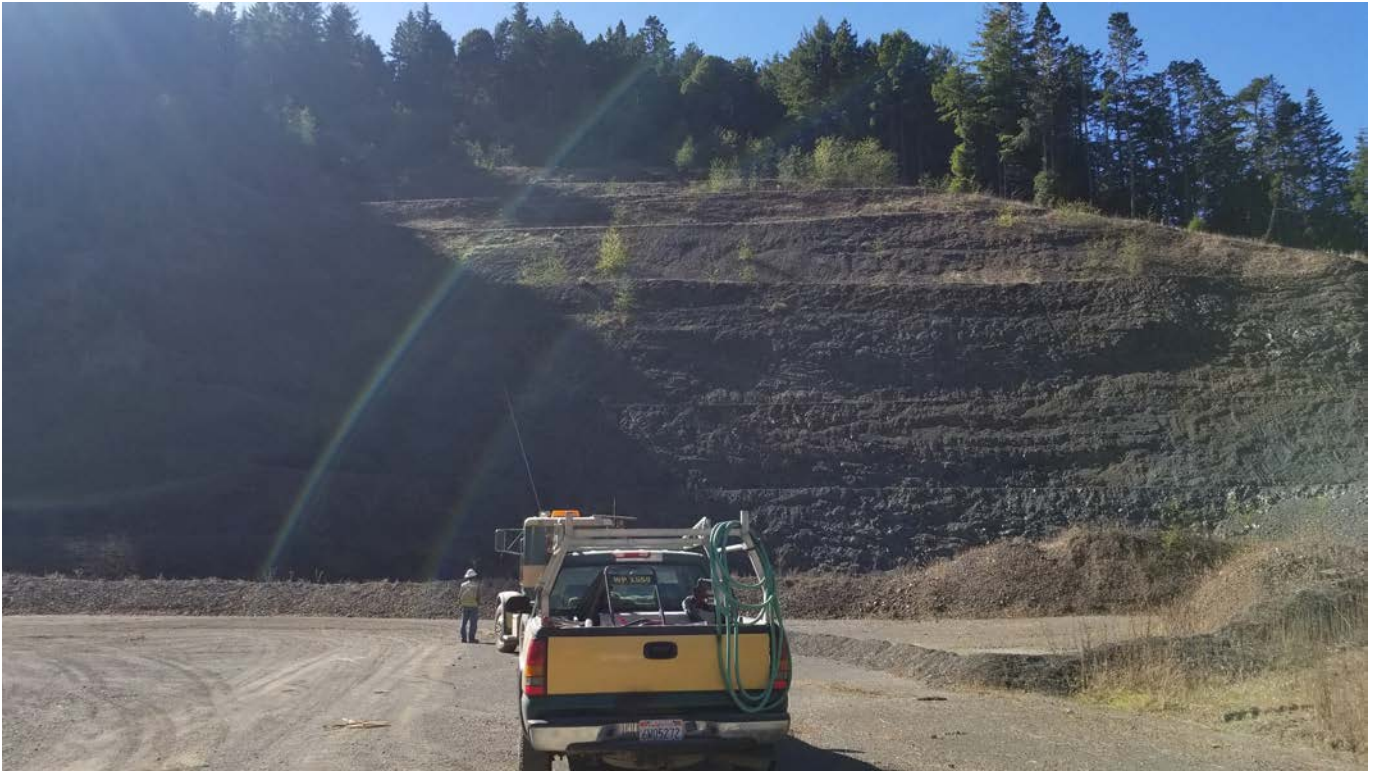
Photo #1 - View from quarry floor, looking southwest. Quarry face with multiple benches, and some vegetation on upper section observed.
