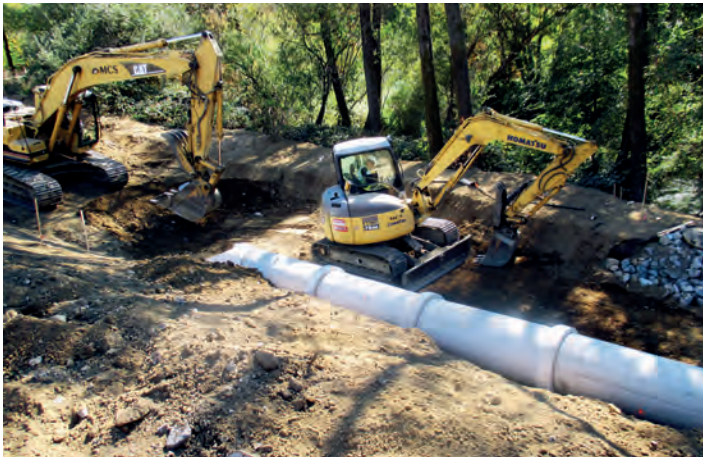
Mendocino County Department of Transportation Heavy Equipment Operator crew working on a culvert replacement project.
