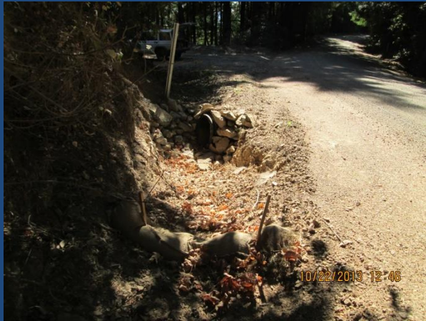
Installation of additional ditch relief culverts
