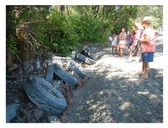
Figure 4. Truck tires cabled together to stabilize the banks of Town Creek. June 7, 2016.
