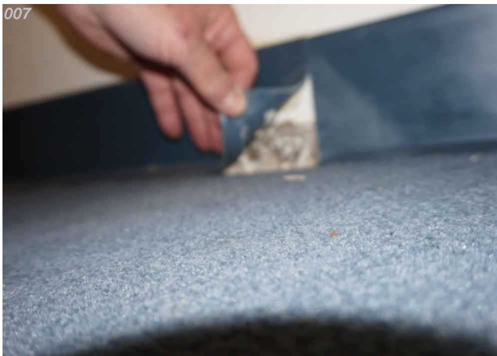
Office 369, Microbial growth behind base coving on South wall
